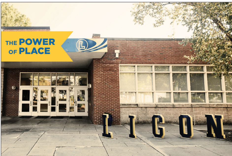
J.W. Ligon Magnet Middle School will be demolished.
